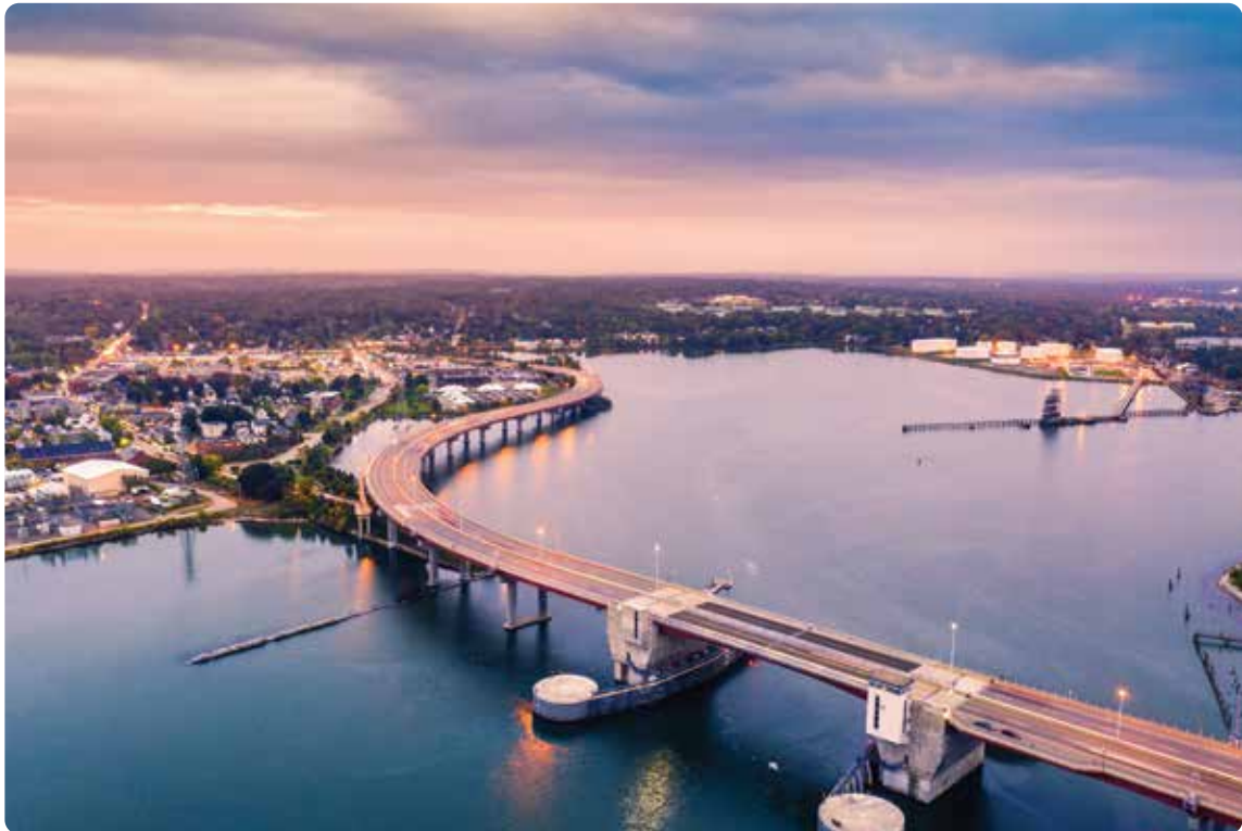
Casco Bay Bridge, Portland
