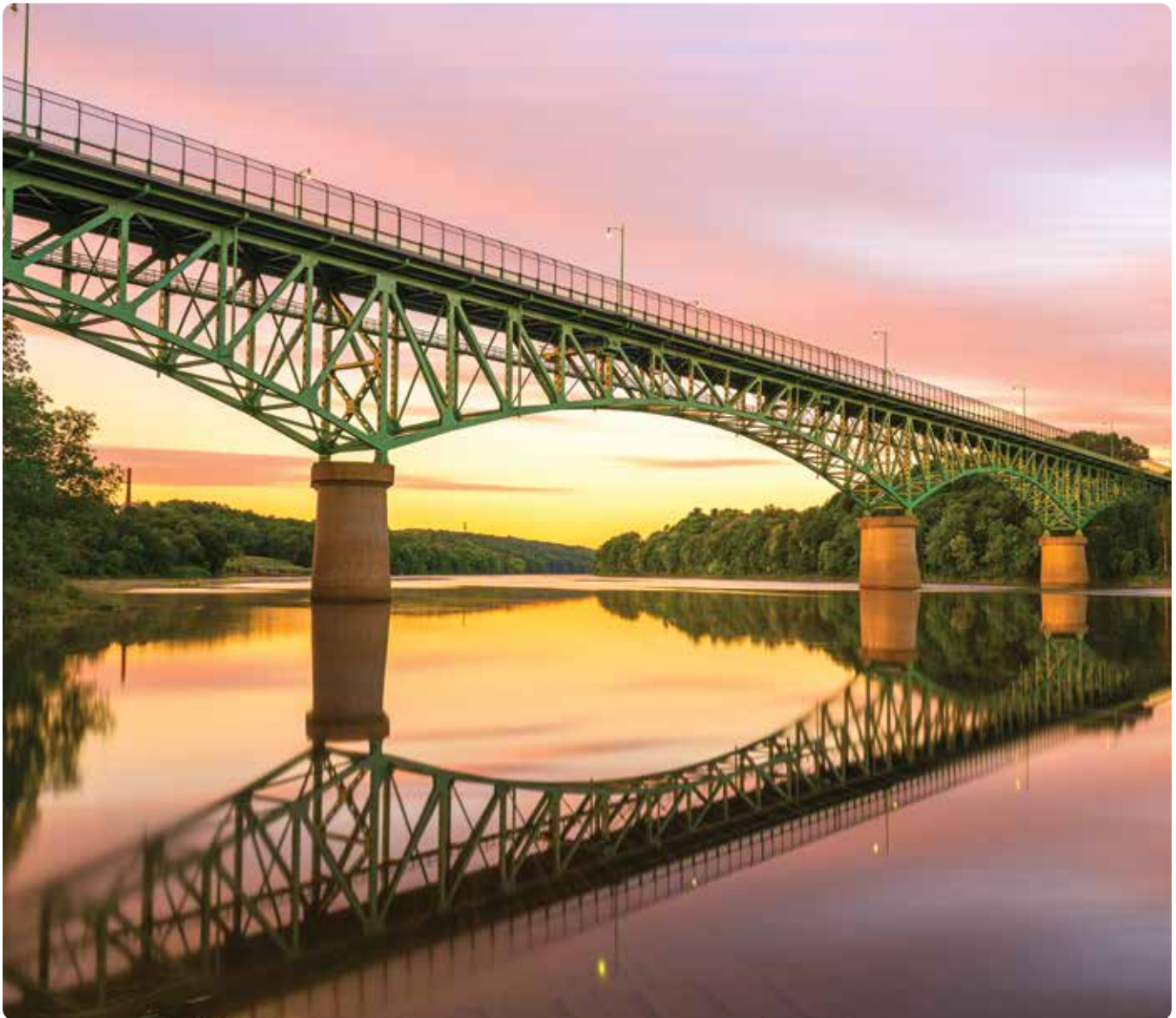
Memorial Bridge, Augusta
