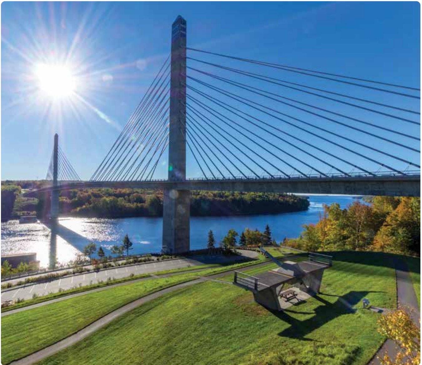
Penobscot Narrows Bridge, Stockton Springs
