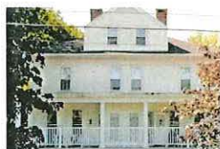
Treasure House at Harbor Place 6 Units 80A High Street Belfast, Maine
